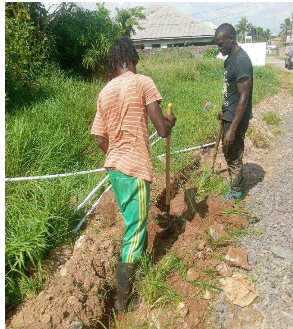
Figure 14. Right: Leaks repair by Technical Services
