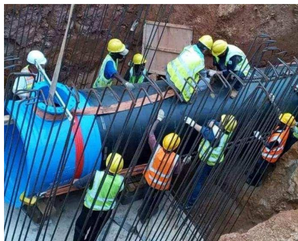
Figure 17. Right: Installation of new 48-inch main pipeline
