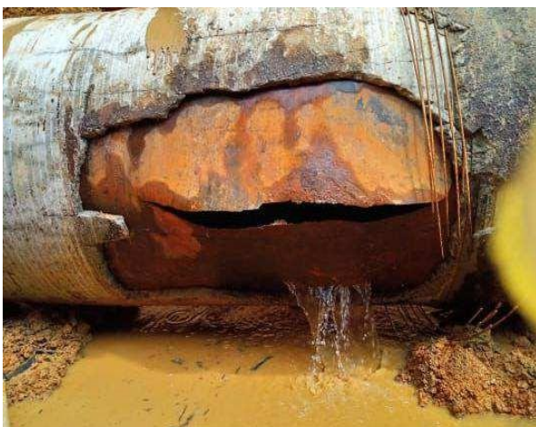
Figure 16. Left: A repair of ruptured 36-inch transmission line
