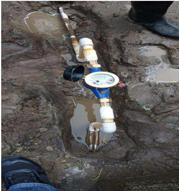
Figure 13. Left: Pictorial view of meter connection
