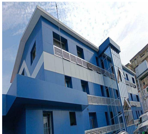
Figure 10. After renovation of Head Office
