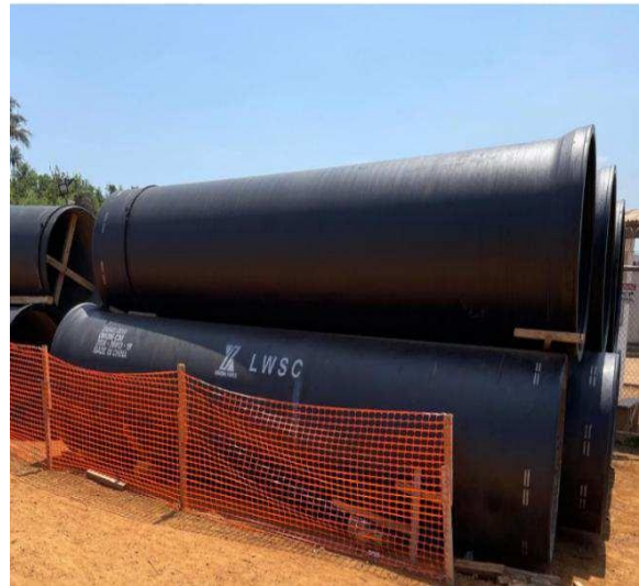
Figure 19. Right: Arrival of 48-inch pipes at project site
