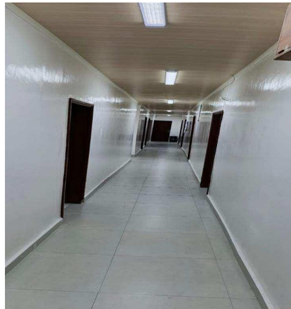
Figure 12. After renovation of Head office
