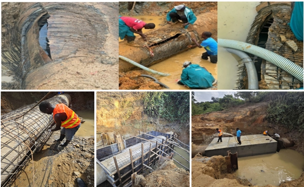
Figure 5: Repair of 36-inch transmission and distribution main
