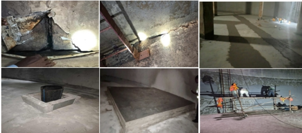
Figure 9: City Reservoir repair works, 2024
