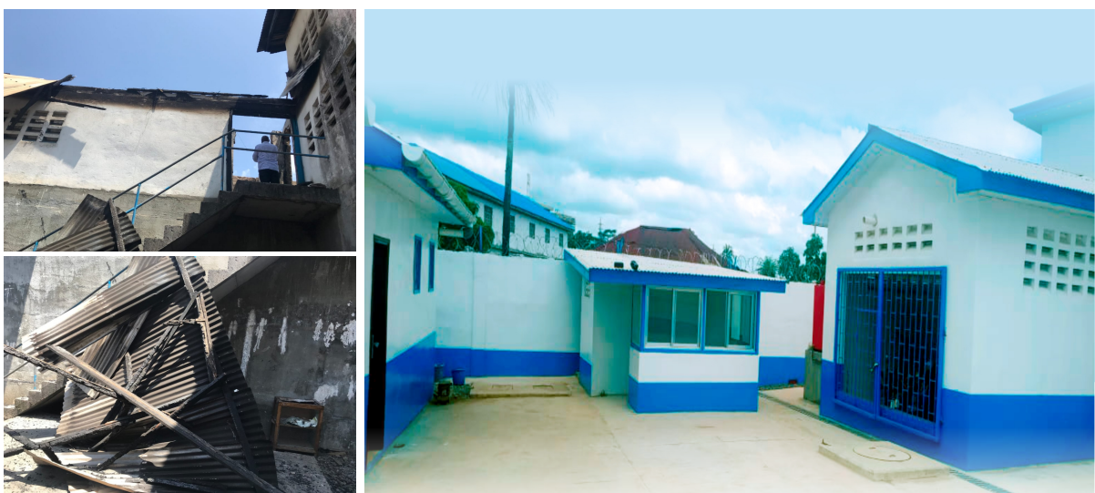
Figure 8: Burnt & reconstructed Caldwell Water Booster System
