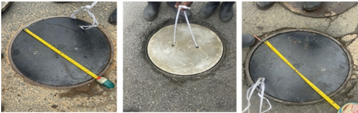
Figure 7: Manhole covers for Sewer Inspection holes
