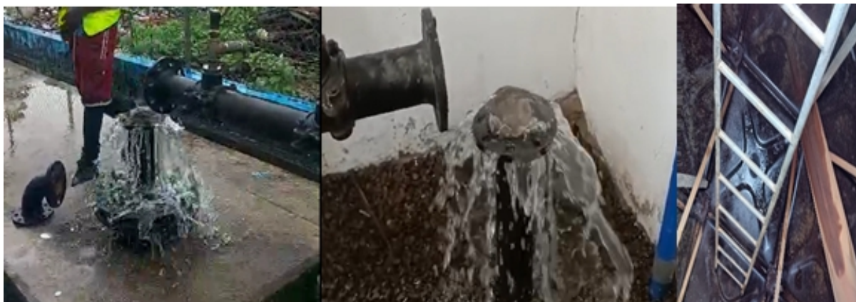
Figure 10: Repair work at Soul Clinic Reservoir
