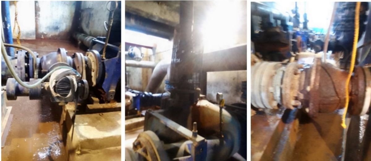
Figure 4: WTP equipment repaired by the Technical Division, 2024
