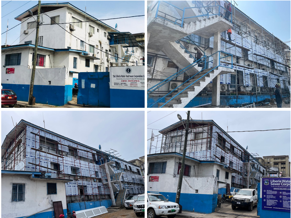
Figure 3: Ongoing Rehabilitation Work on the Corporation's Central Office
